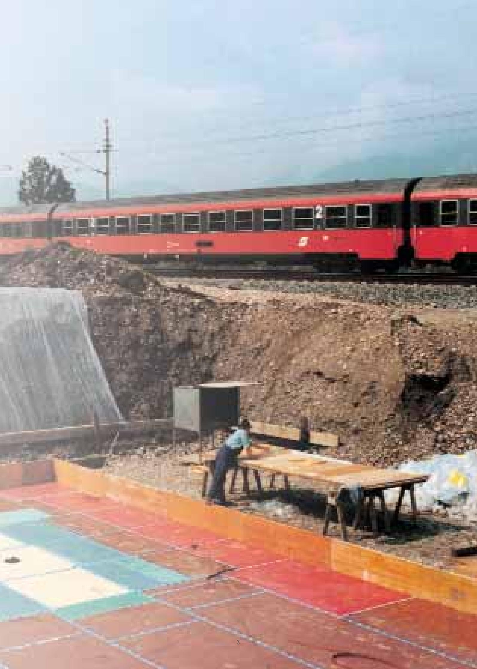
With Sylomer®, the designer has a technical material available for resilient bearing purposes, which suits a multitude of construction methods. The bedding can be provided over the full surface, in strips or at individual bearing points. The specific location at which the building must be resiliently separated is not predetermined for a bedding on Sylomer®. Separation is made wherever it is most favourable for the design.
