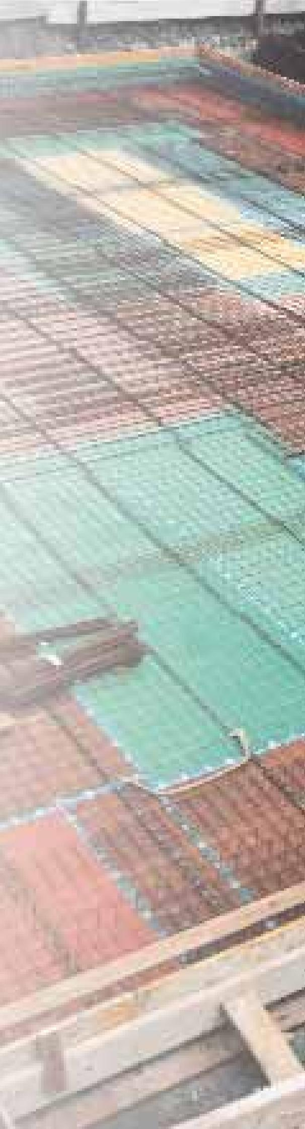
The bedding on Sylomer® can be full surface, on strips or on point bearings. The bearing design for the building depends on the specific natural frequency and the construction features. Connecting structures, such as ceilings or walls, can be of in-situ concrete or can be prefabricated. When cast from in-situ concrete, the bedding surface is normally utilized as lost formwork. The reinforcement can be fitted directly on the mats. For
