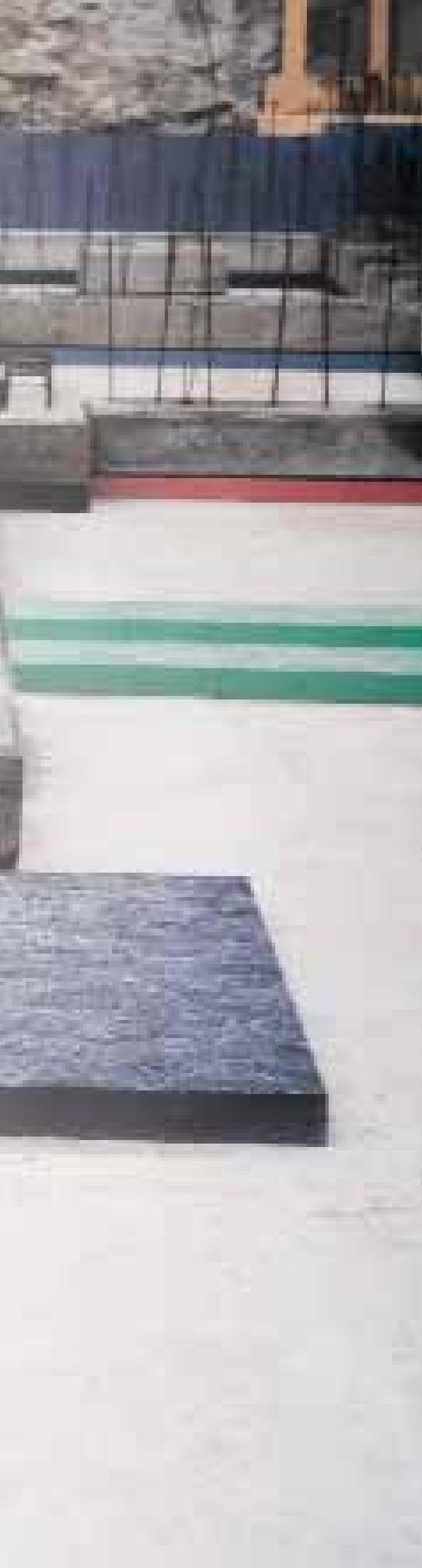
**S**ylomer® bedding is supplied to site in sheets or cut to size as individual bearings. Cutting on site is possible with standard tools.
