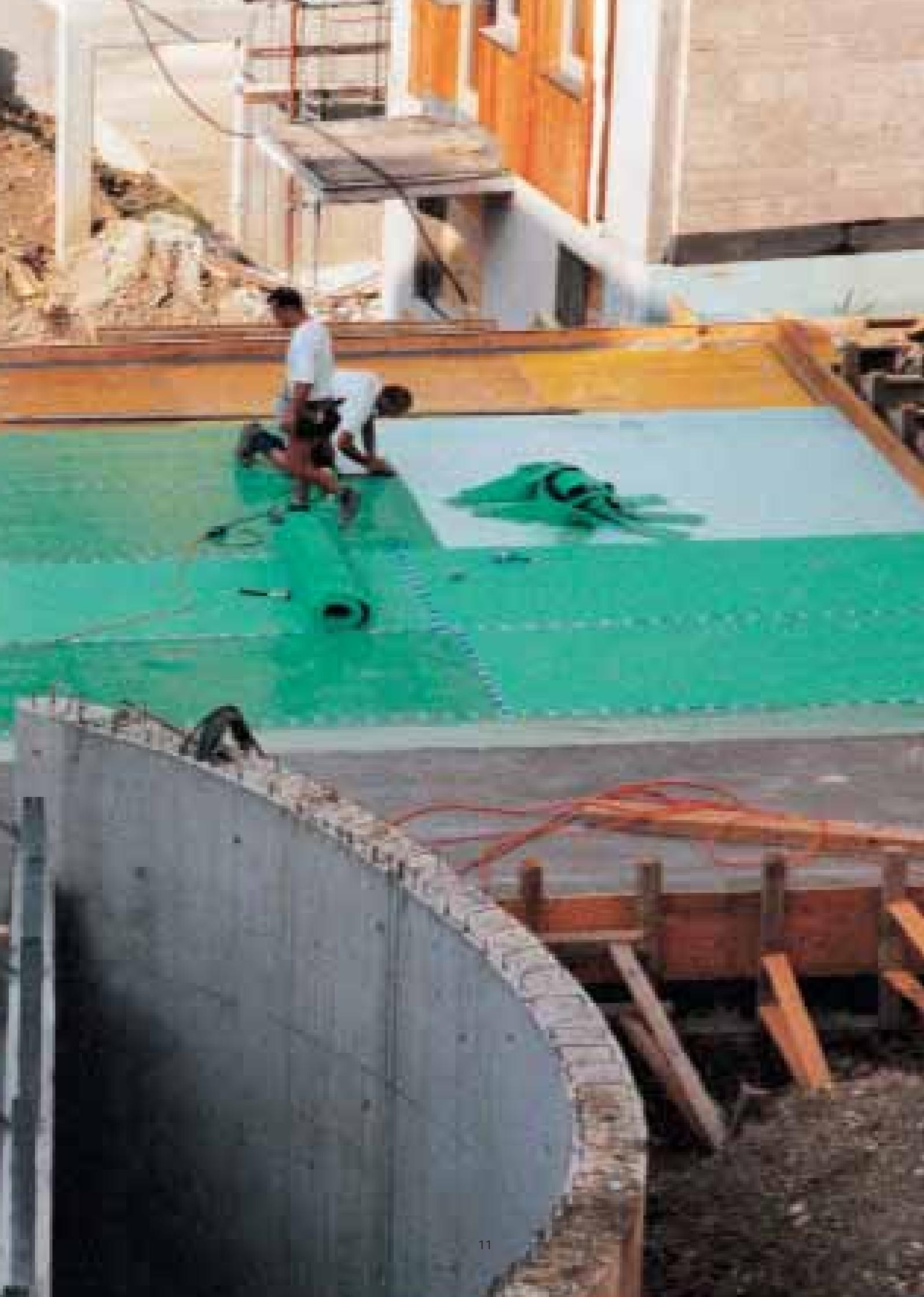
**S**ylomer® sheets and the bearings they form, are flexible and adapt to the contours of the foundation when loaded. The stiffness of the bearing depends on the load it supports and increases with this accordingly.
